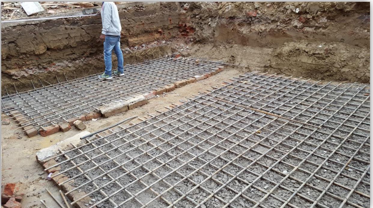
REBARS CHECKING FOR RAFT FOUNDATION
