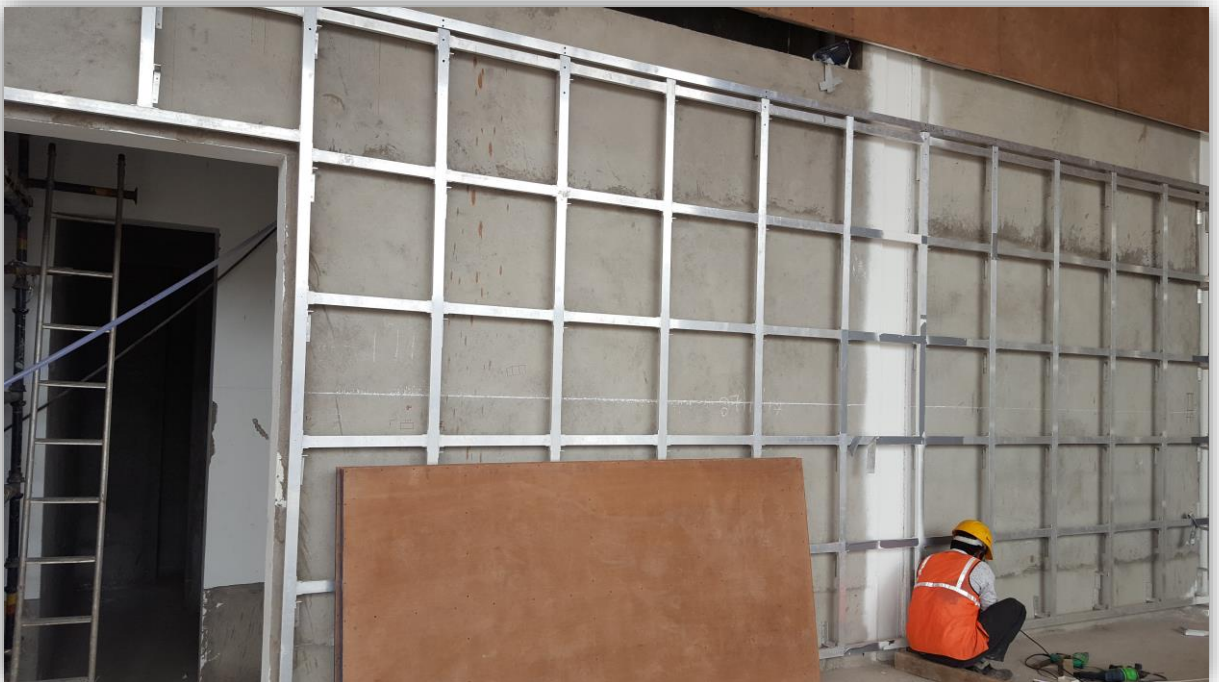
ONGOING INTERIOR AT CAFÉ CUM RESTAURANT AT RANCHI
