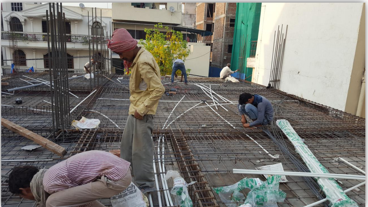
BRICK MARKING & CONDUITS MARKING CHECKING
